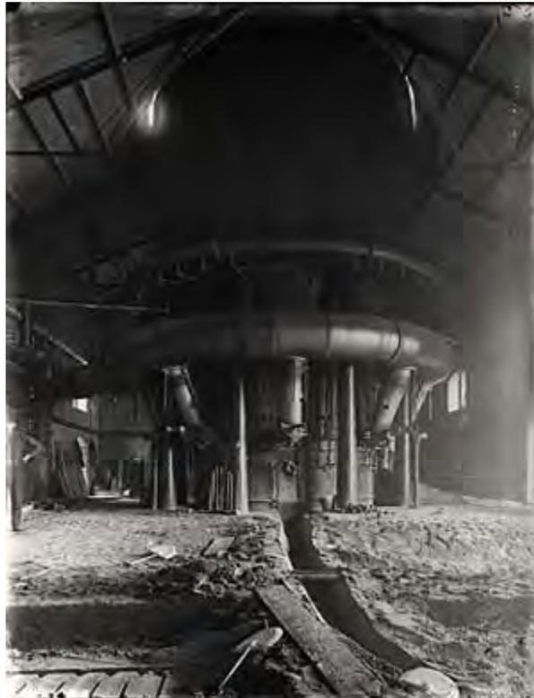
Blast furnace at Canada Iron and Furnace Co. Midland c.1900
